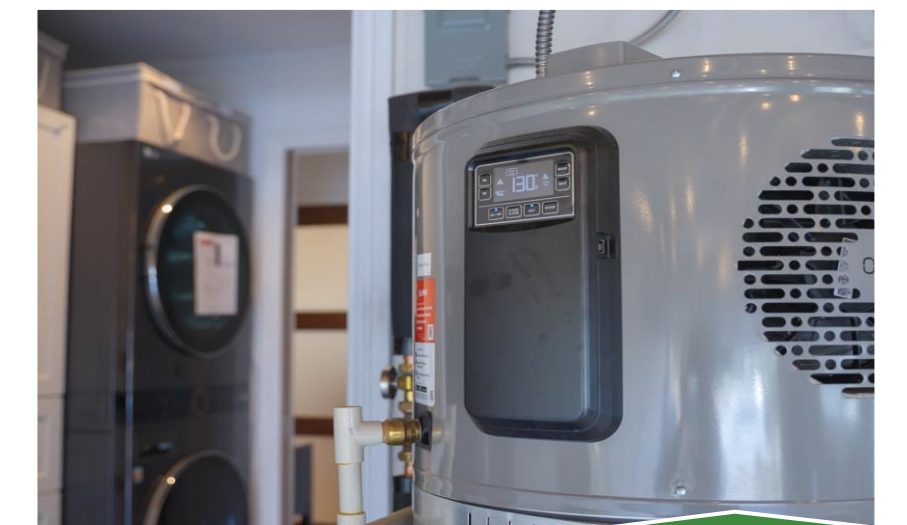
Emergency Water Heater Replacement
