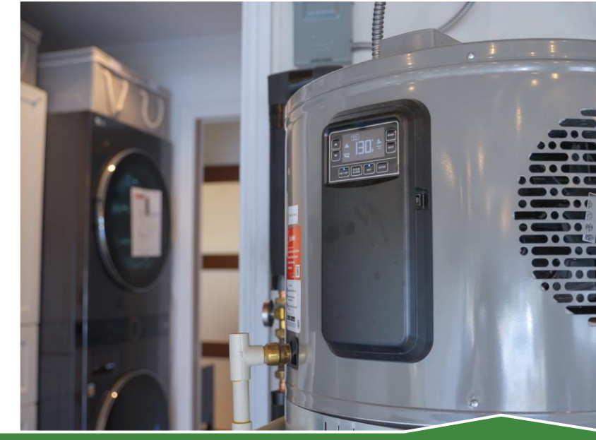
Emergency Water Heater Replacement
